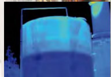
Tank level too low
